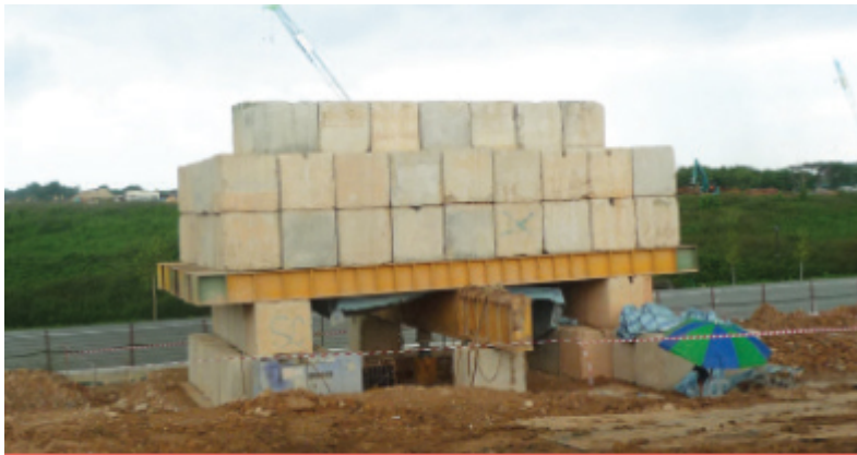
Kentledge pile loading test with concrete blocks
